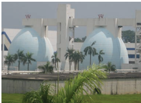
■ Figure 19.13 Waste water treatment plant in Singapore (currently ultrafiltration and ultraviolet radiation, but microbial fuel cells are under investigation at the National University of Singapore)
