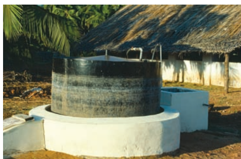
■ Figure 10.61 A small-scale biogas generator uses animal waste to produce methane for a village's needs.
