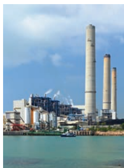
■ Figure 8.29 An oil-fired power station
