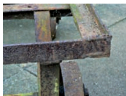
Figure 9.2 A rusting railway trolley (showing pitting)
